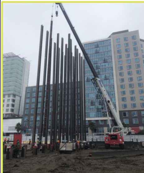
Block A piles
