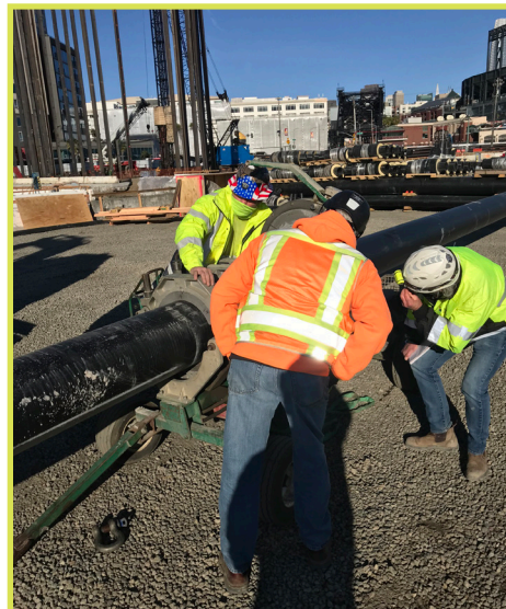
Start of utility piping connections
