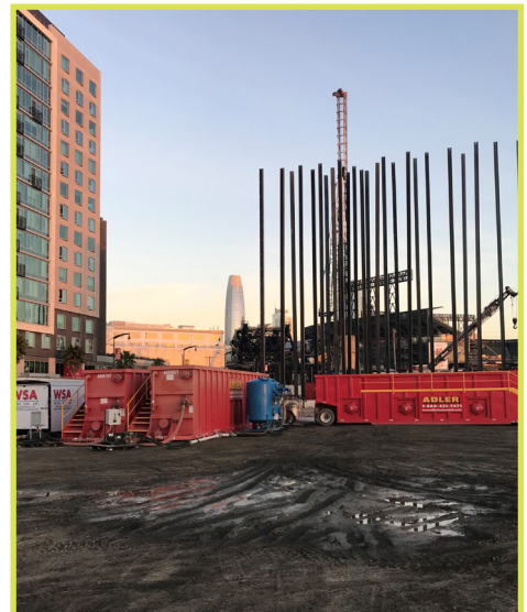
Start of Third Street dewatering system
