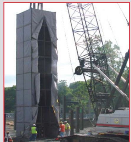
Noise Mitigation Method – Shroud on Rig Hammer
