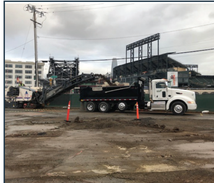
Pavement grinding
